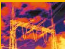
Inspection of high voltage power lines
